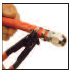
2 Crimp with clamp pliers.
